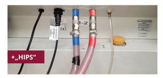
5. Check the water connections and condensate hose for tightness and correct seating. Red to red and blue to blue.
